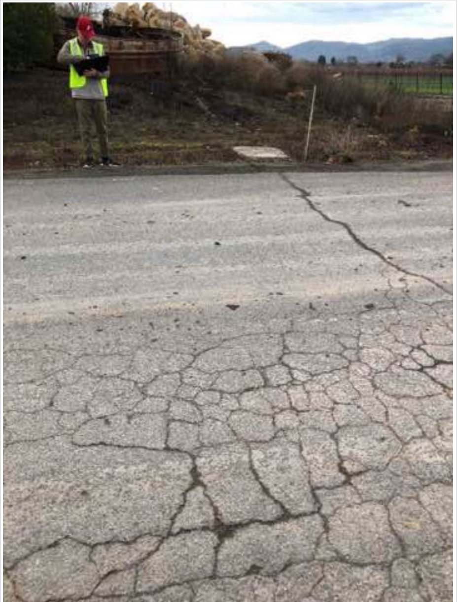
Photo Showing Reference Point (Measure Distance) to new pole
