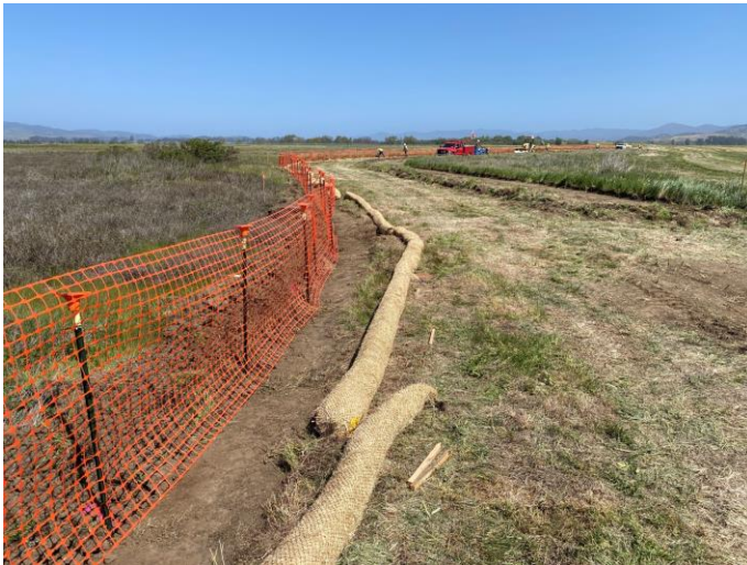
Install erosion control
