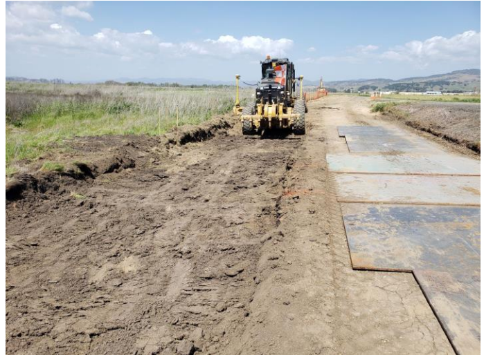
Service road earthwork activities
