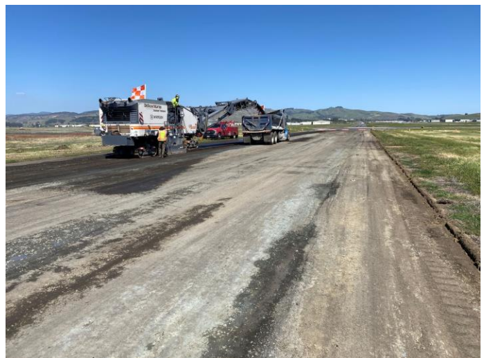
Remove taxiway pavement
