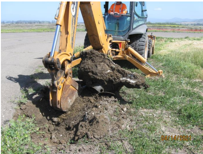
Remove taxiway lights
