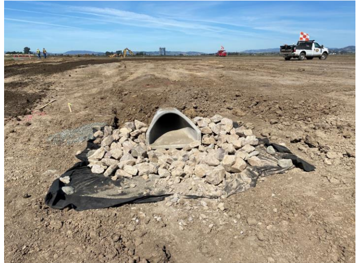
Flared end section and riprap installed
