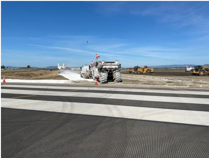
Lime-treat taxiway subgrade
