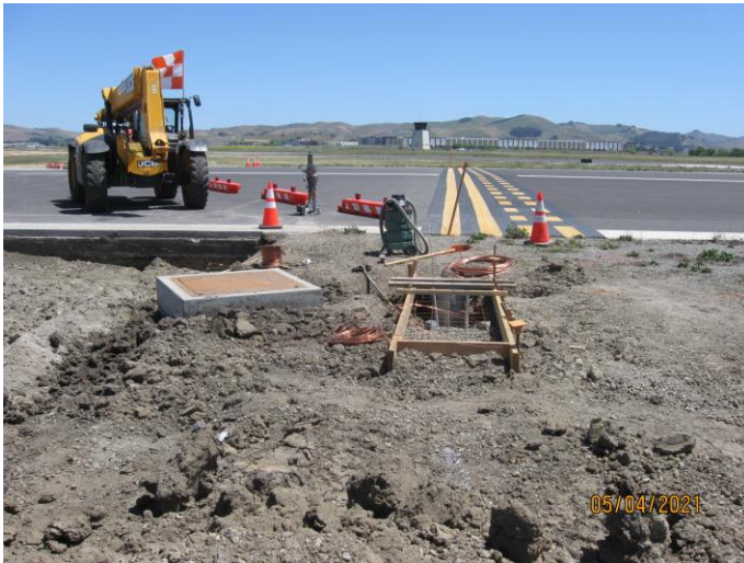
Sign base formed next to pullbox
