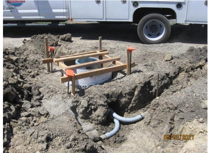
Forming junction can installation
