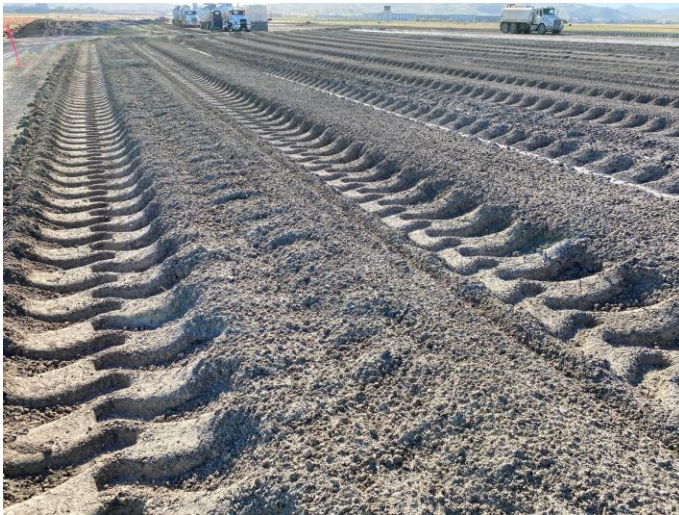
Lime-treating new runup apron
