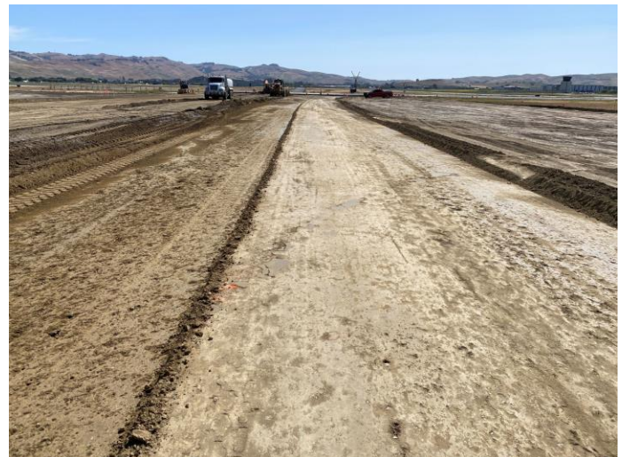
Finish grading Taxiway H lime-treatment
