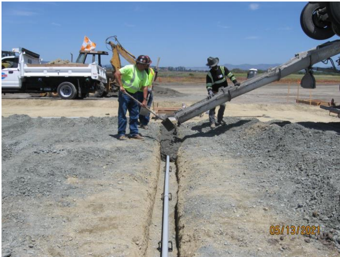
Backfill electrical trench across Taxiway H
