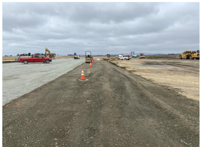
Compacted recycled base on taxiway shoulder
