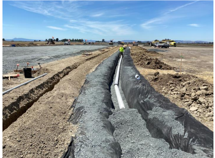
Underdrain and electrical trenches along shoulder
