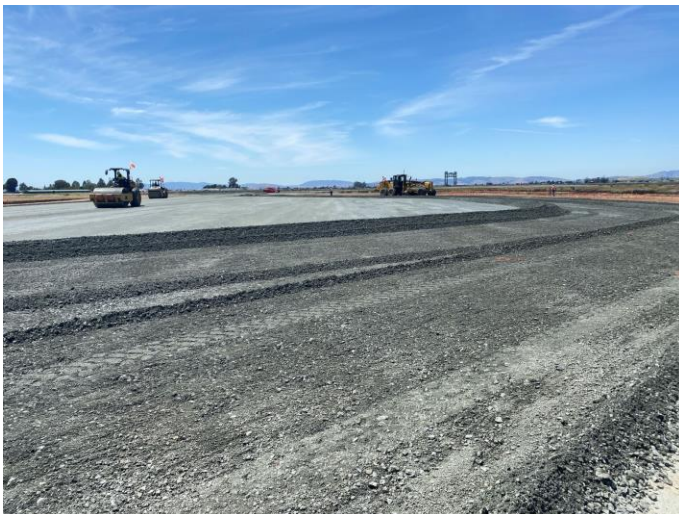
Placement and compaction of P-209 aggregate base
