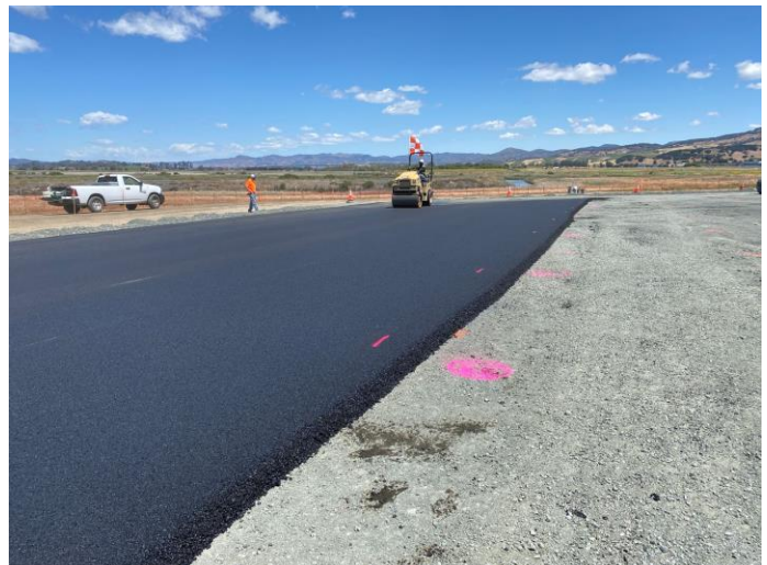
P-401 asphalt control strip on runup apron
