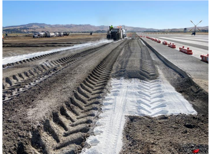
Lime treatment in Work Area 4
