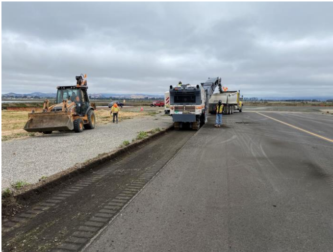
Pavement removal in Work Area 4
