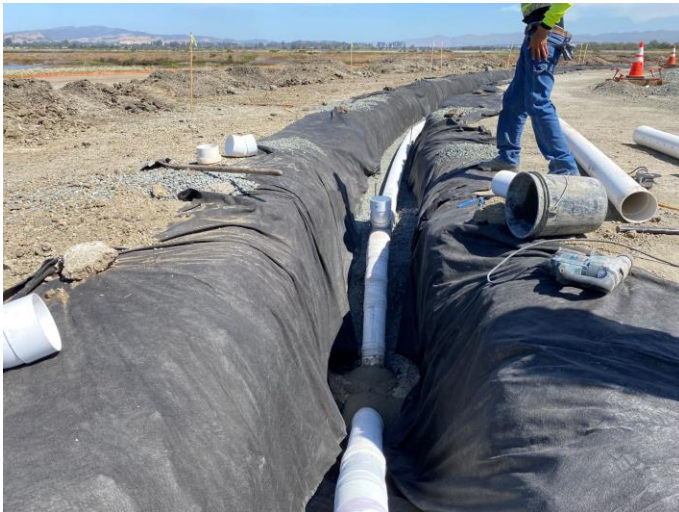
Underdrain connection to new storm drain culvert
