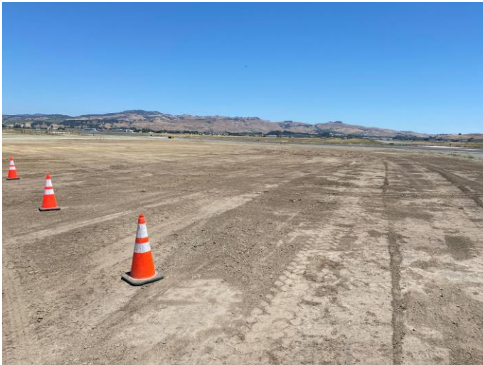
RSA graded at runway intersection
