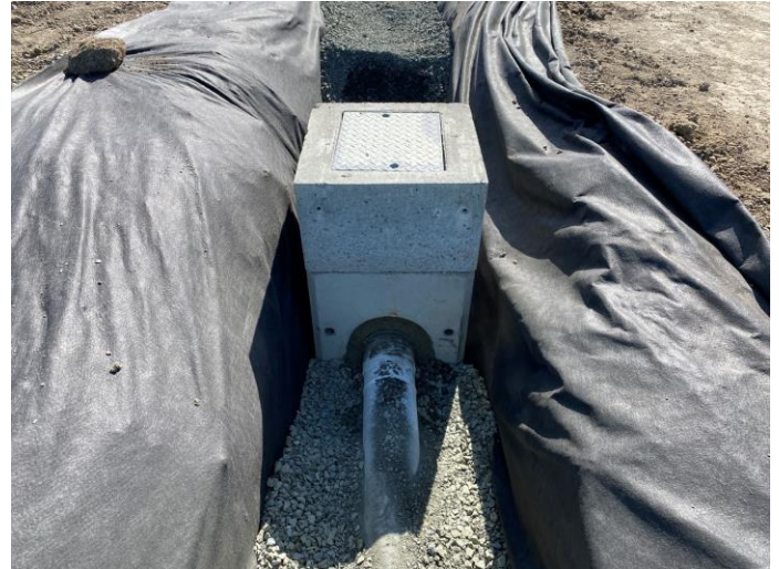
Underdrain connection to new catch basin
