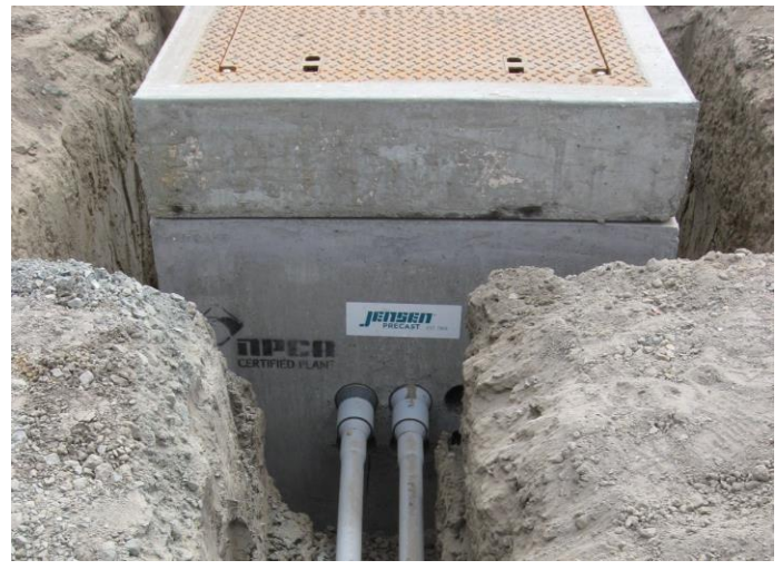
Conduit connection to new electrical pullbox
