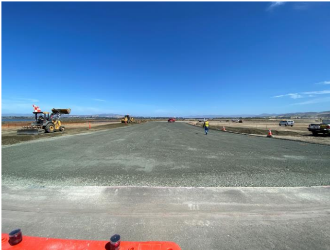
P-209 AB finished in Work Area 4
