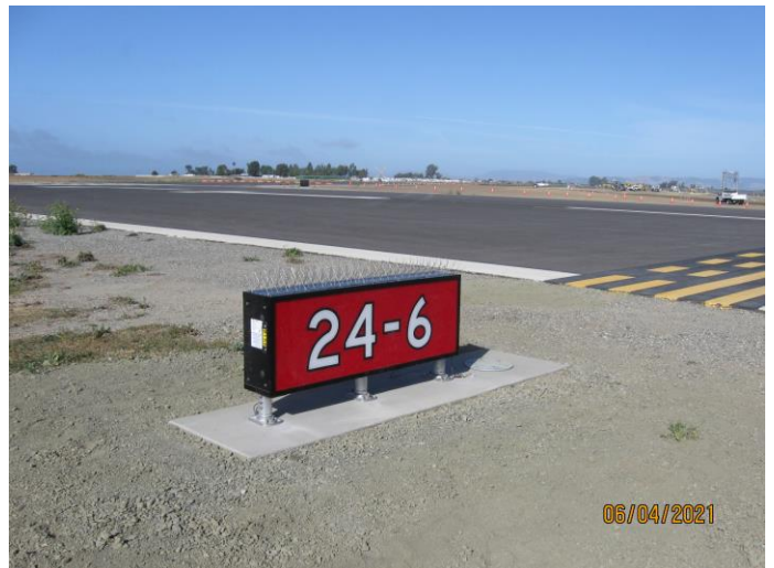
Runway holding position sign installed
