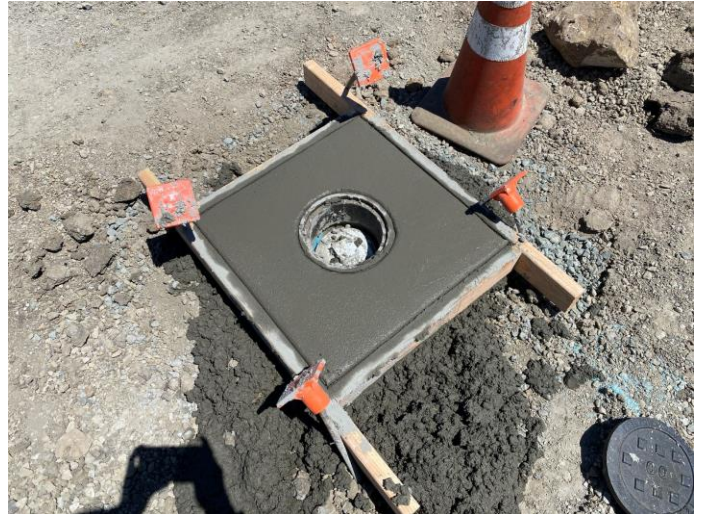
Concrete poured in underdrain cleanout cover
