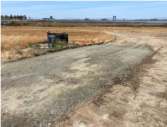
Service road constructed to REIL
