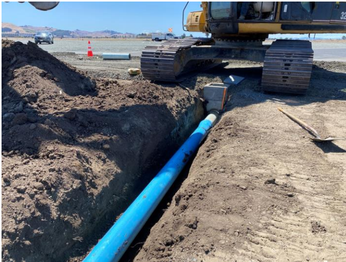
Installing underdrain outflow pipe
