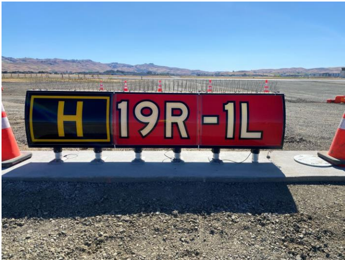
Runway holding position sign installed
