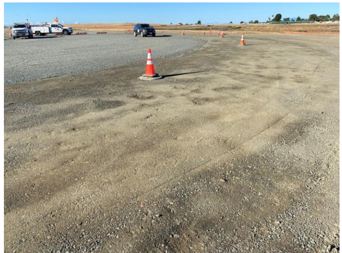
Compacted taxiway shoulder base
