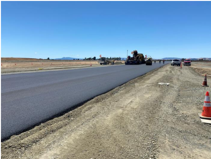
Paving Taxiway H
