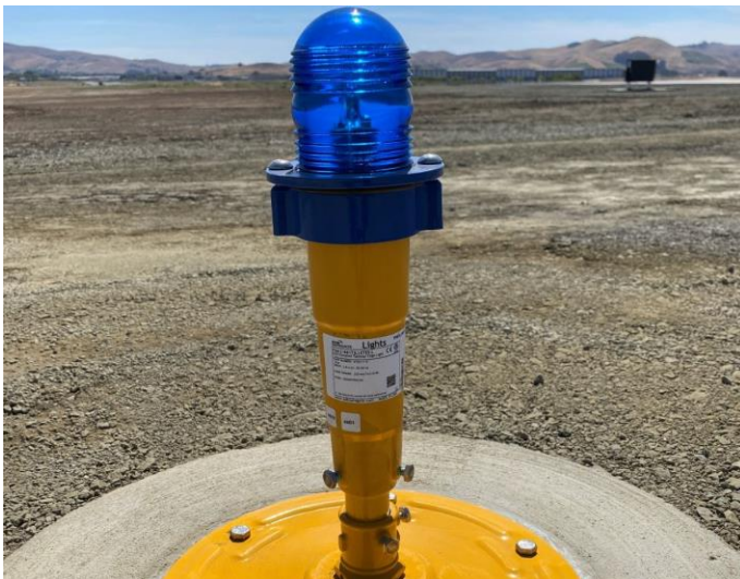
Elevated taxiway light installed
