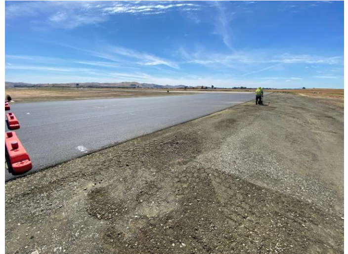
Finishing Taxiway H shoulders
