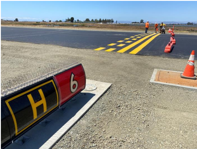
Runway 6 holding position markings and sign
