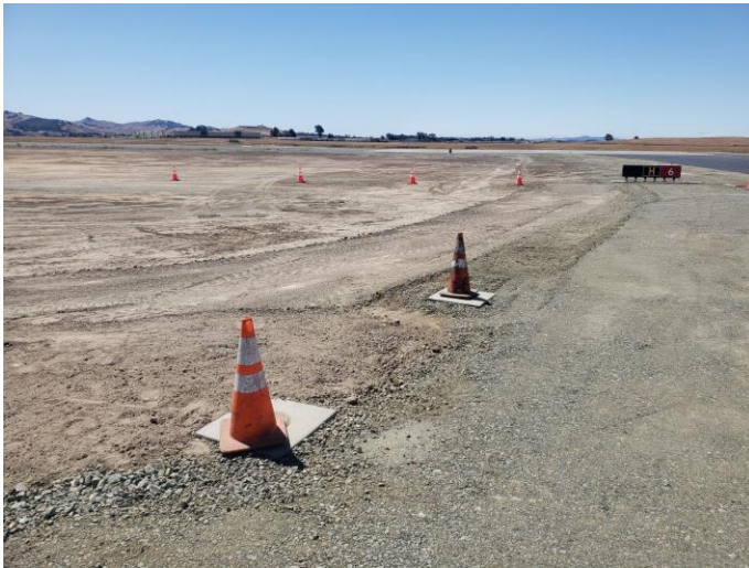
Finishing safety areas beyond shoulders
