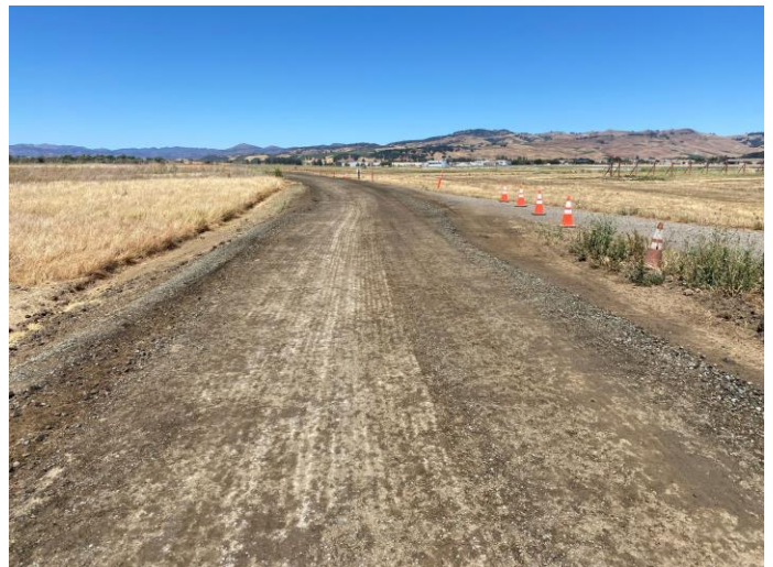
Finishing service road
