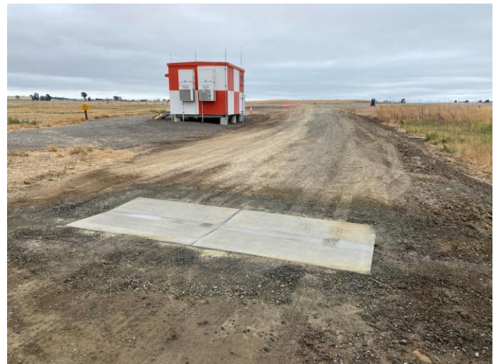
Finished valley gutter
