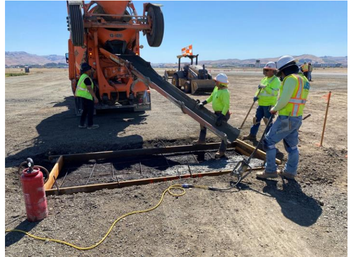
Valley gutter formed and being poured
