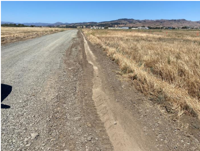
Finished service road with flow line
