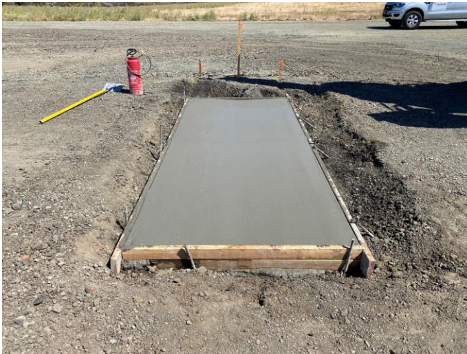
Valley gutter poured and curing
