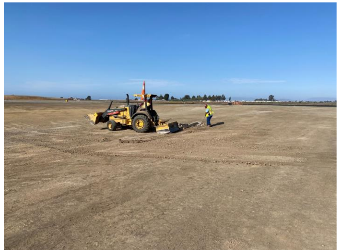
Final grading of infield flow line
