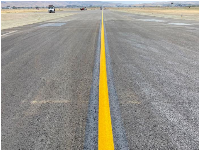
Taxiway centeline marking complete
