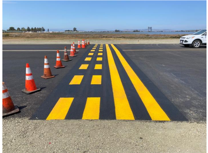
Runway holding position markings complete
