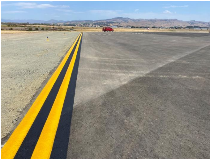
Runup apron markings complete
