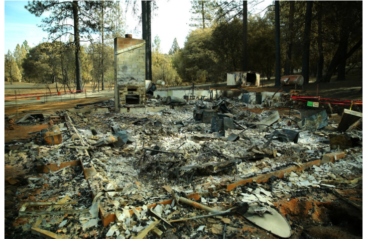
The 2015 Butte fire in California scorched 110 square miles of public and private property, including this single-family home. Over 549 homes were burned down to the ground as a result of fast-moving wildfires that were catastrophic to this community. Photo by Adam DuBrowa/FEMA
